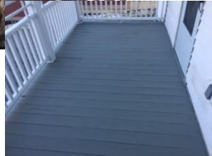
Rot Repair at 10 S Water St
