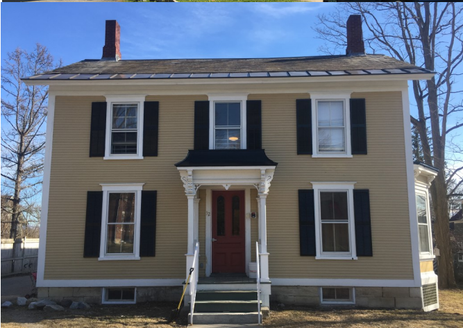
Above: 32 Seminary St in Middlebury before and after new railings and trim, landscaping, and a fresh coat of paint.
